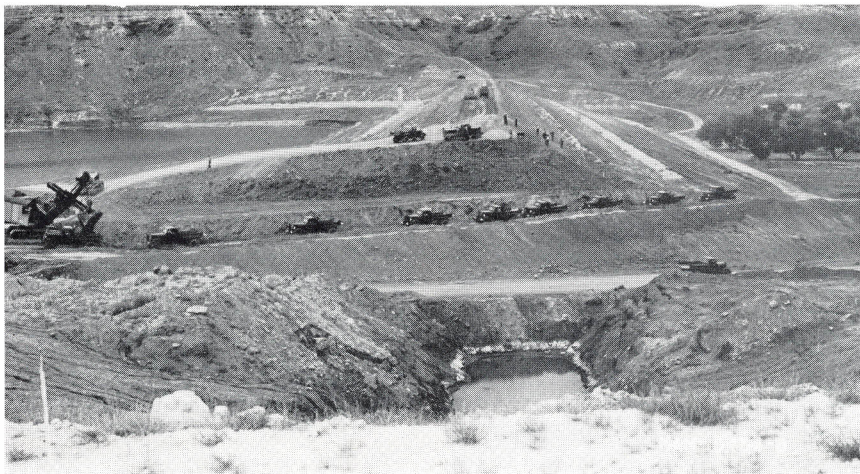
This photo, taken in the 30's, shows the construction of the dam and spillway. It was the largest dam in Kansas at this time.
