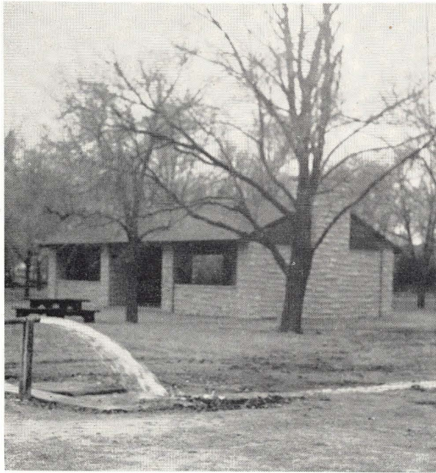
The new shelter house at the north end of the lake nestles in a grove of trees. An artesian well seen in the foreground is three-hundred feet deep and flows at the rate of 100 gallons per minute.
